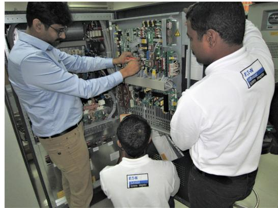
Major PM Visits will require that the UPS be put into “bypass” and isolated so the UPS can be safely inspected including its internal components. See UPS below.
