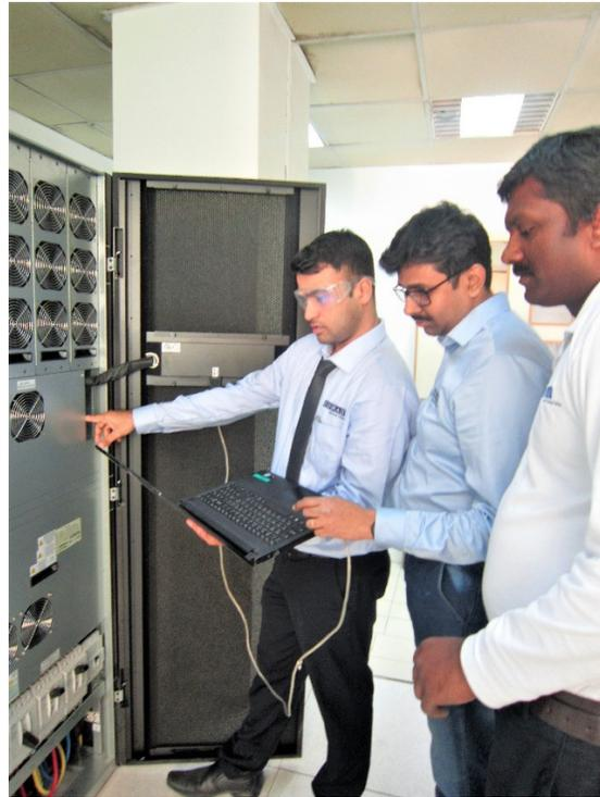
We will vacuum and/or blow out dust and debris, inspect air filters and replace as necessary. Close inspection of capacitors will occur with meter testing where deemed necessary. (Sencore LC53 capacitor-inductor meter) All cables and connections will be inspected and checked for tightness and re-torqued where necessary. Seating of components and control wiring is checked.
