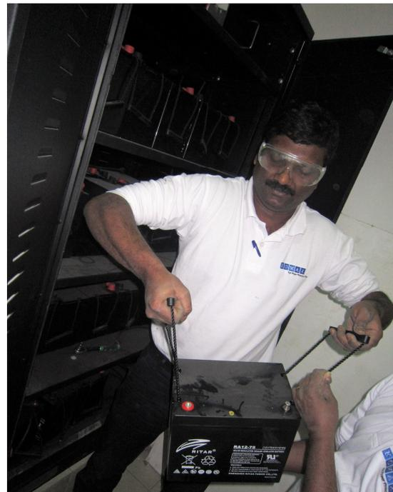
Anything 8 VDC or less is considered bad and should be replaced soon. 4-8 VDC should be replaced very soon. Less than 4 volts should be replaced immediately, in which case, if a battery isn’t immediately available, we would jump out the bad battery and adjust the float voltage accordingly. (This will depend on how many bad batteries are found and other factors).
